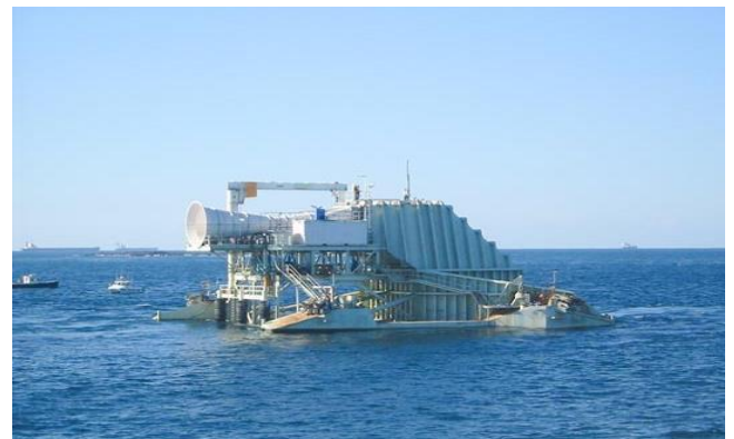
Fig 31:- Oceanlinx 1MW Nearshore OWC Plant
