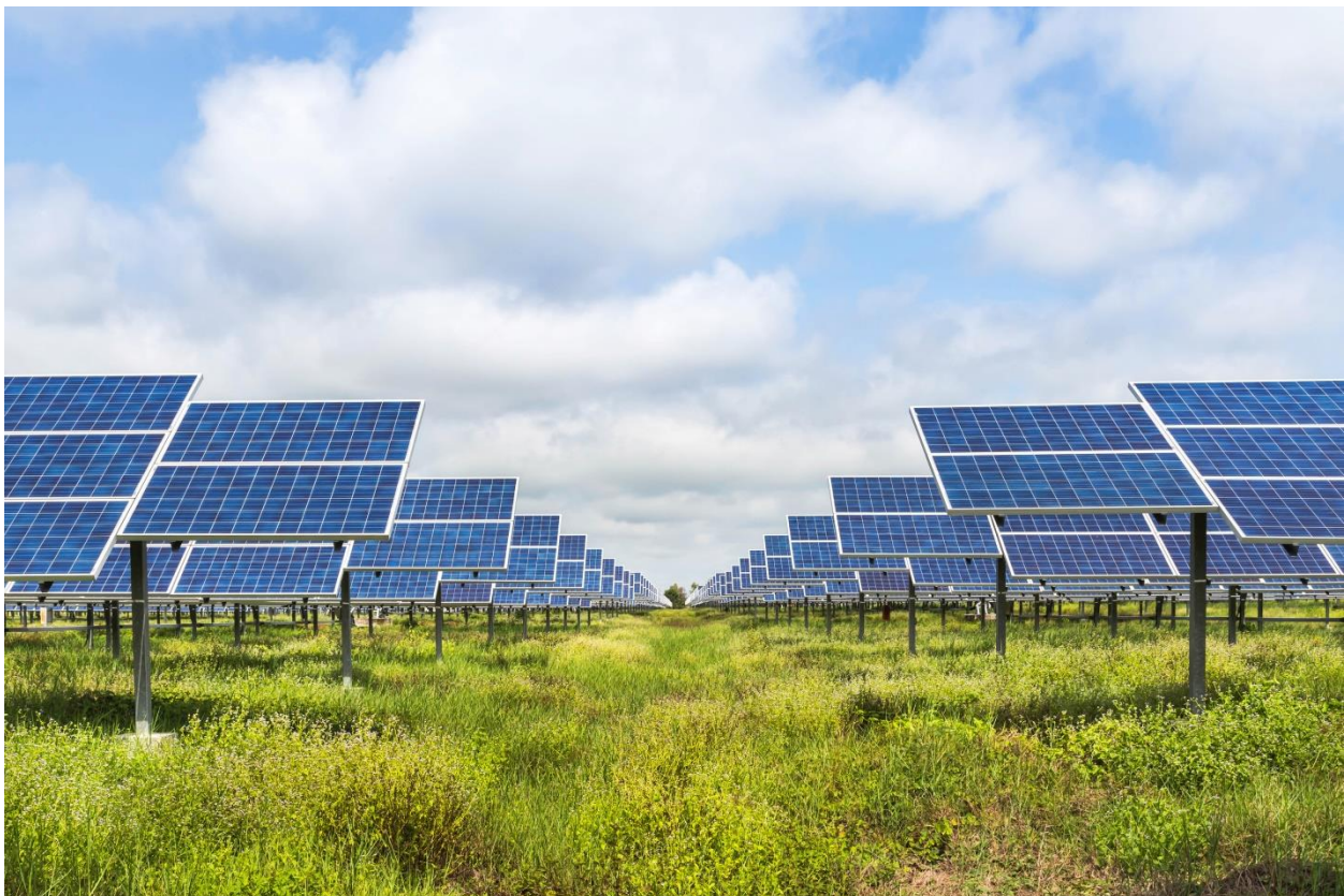
Figure 0-1 Typical solar power system farms
