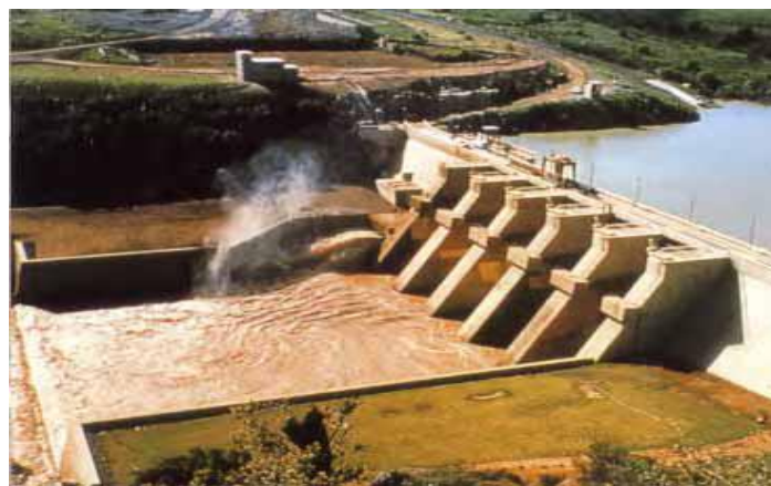
Fig 7:- Welbedacht reservoir during flushing
