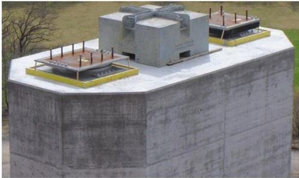
Fig 10: bearing of the bridge
