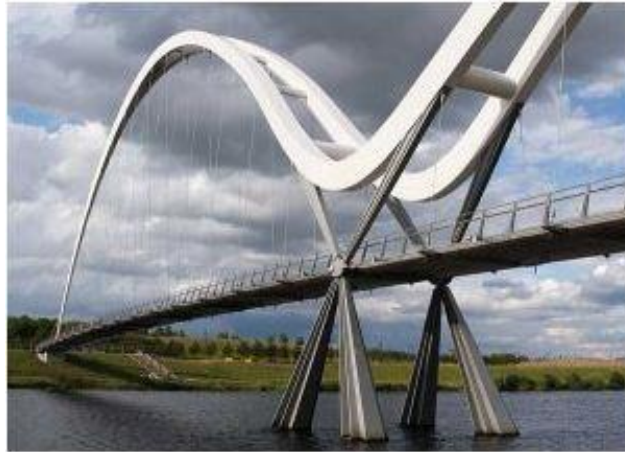
Fig 5: Tied Arch Bridges
