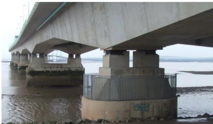
Fig 16: Foundation of Bridges
