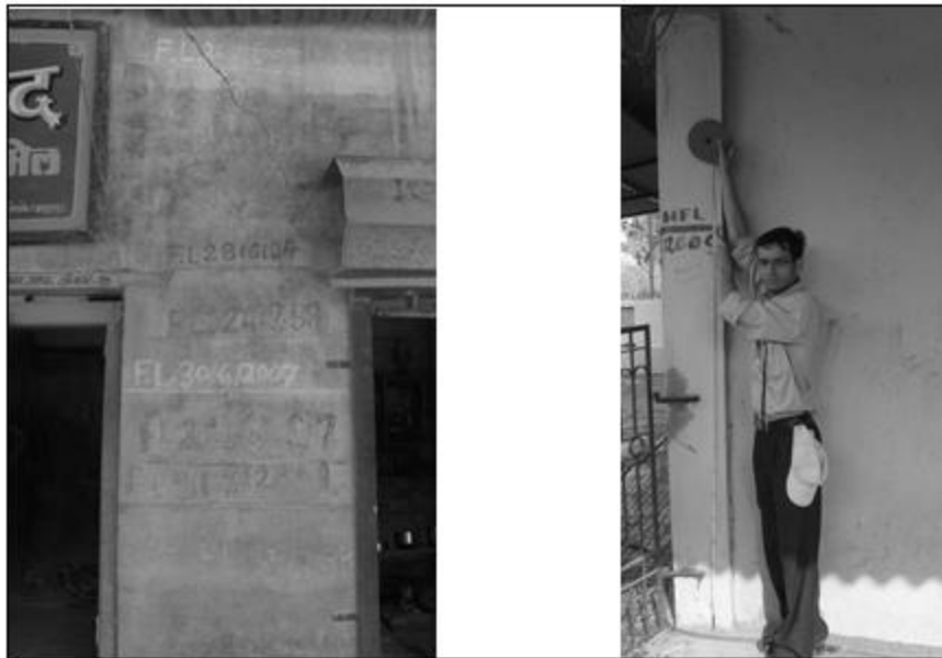
Fig 5:- High Flood Level Markings on the Building Wall
