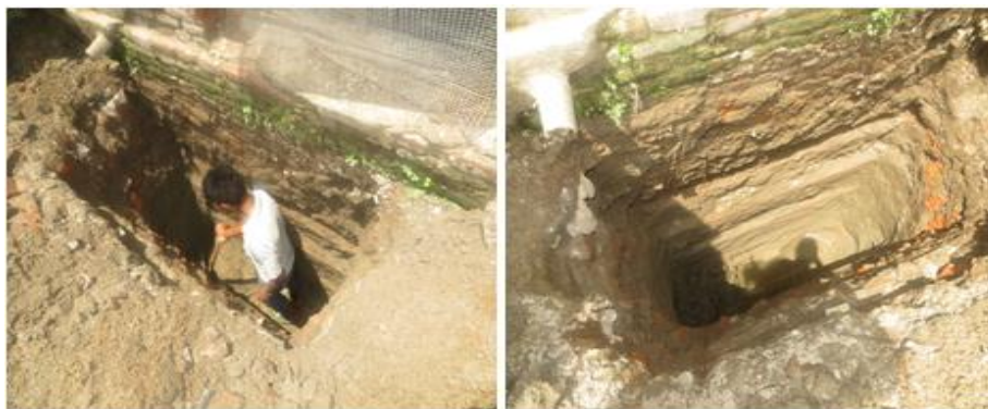
Fig 20:- Foundation Investigation in Charkhal Adda
