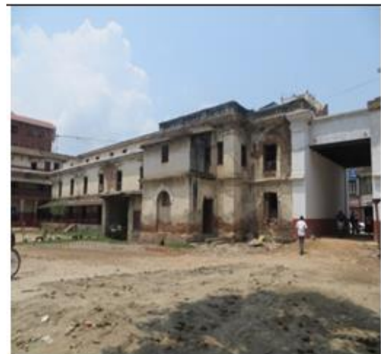
Fig 1:- Front View of the Building
