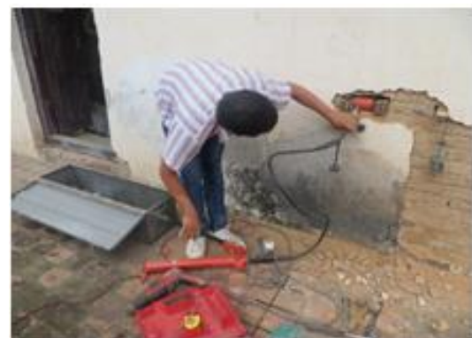
Fig 11:- Shear Test in second floor wall of north wing
