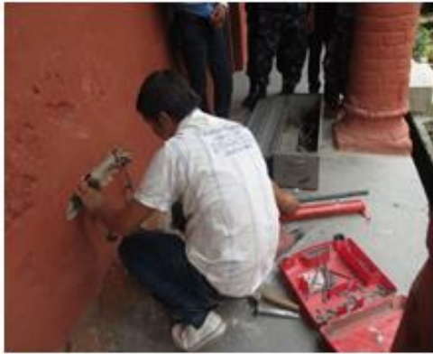
Fig 12: Shear Test in ground floor wall of south wing
