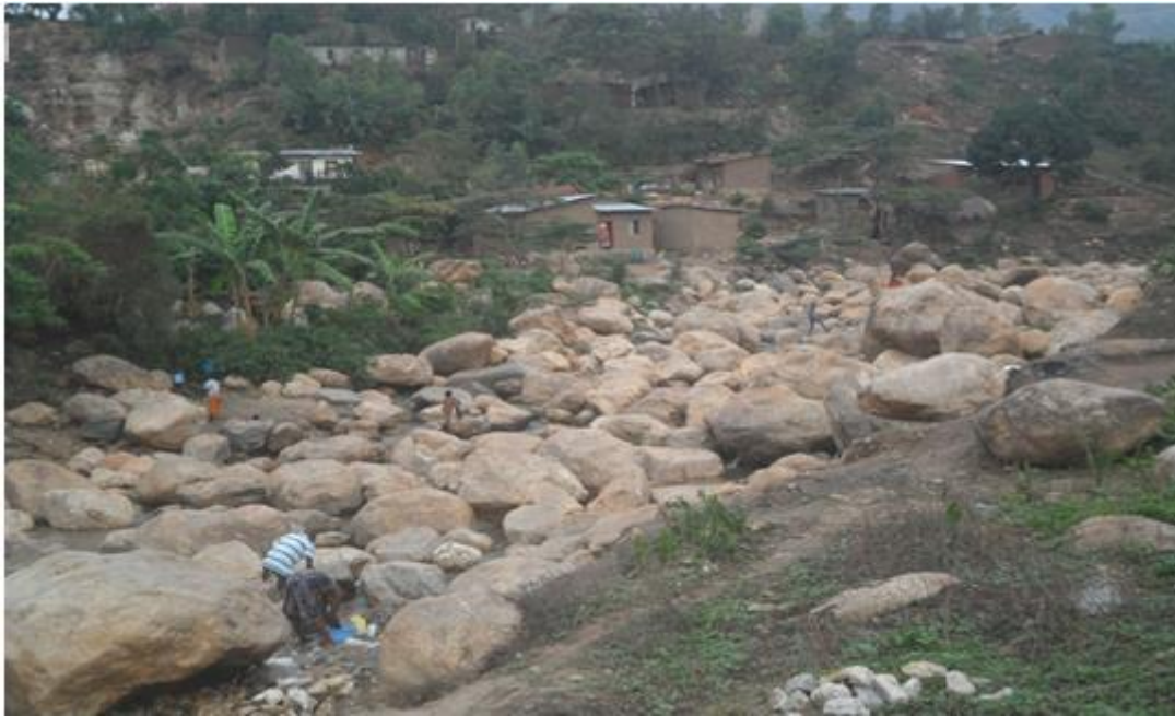
Fig 8:- These houses built on the right bank at the foot of an old terrace.
