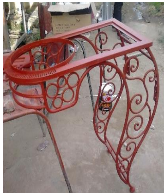
Fig 22:- The application of iron oxide paint (antirust).
