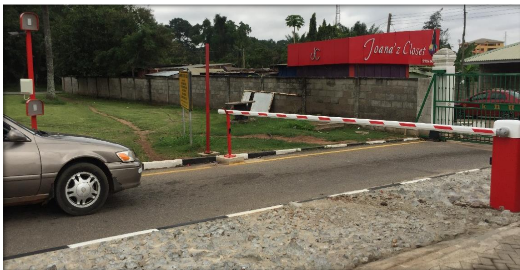
Fig 4:- KNUST electronic vehicular access control system
