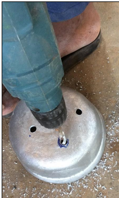
Fig 24:- drilling of conduit holes
