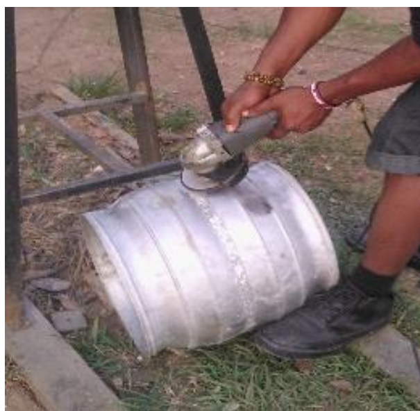
Fig 13:- Grinding of the flux off the frame
