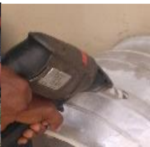
Fig 14:- dilling peg holes
