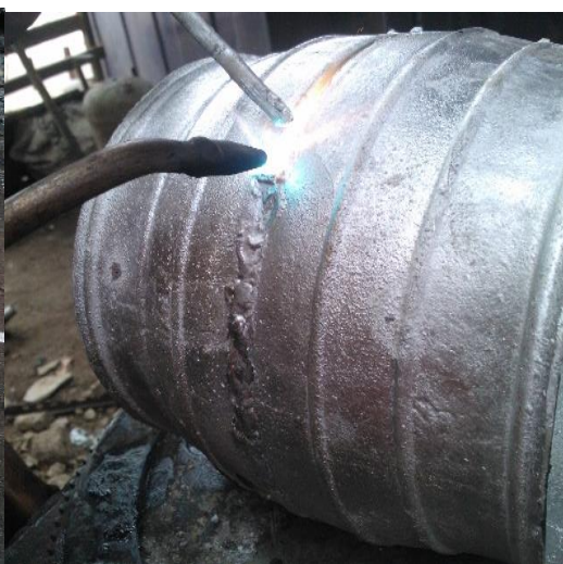
Fig 12:- Welding of the dadesen with gas
