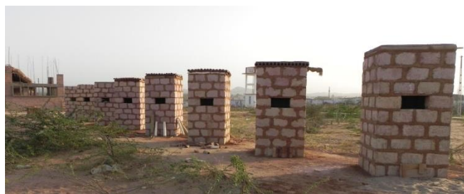
Fig 5:- Modules Constructed on site
