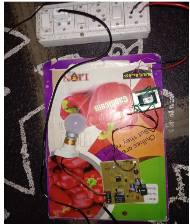
Fig.11. Proposed System when there is an over voltage in AC supply mains
