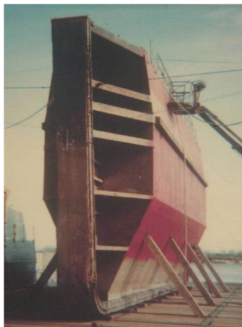
Fig 2:- Graving Dock Gate
