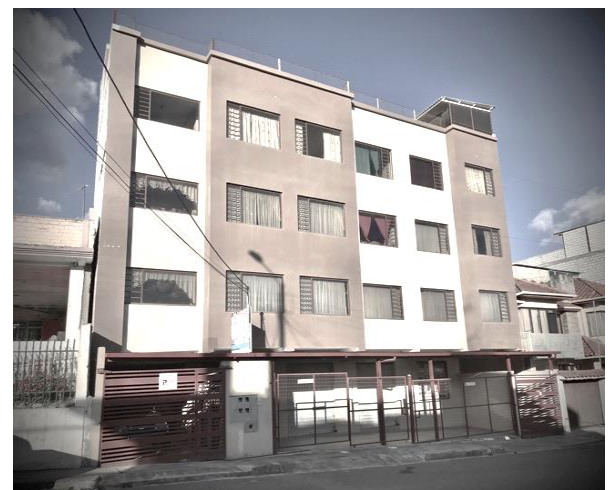
Fig.4. Current state of the building.
