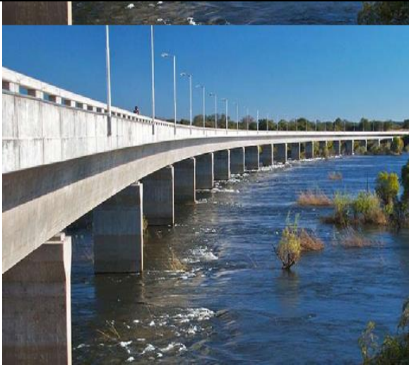
Fig 3:- Mkapa Bridge in Rufiji river
