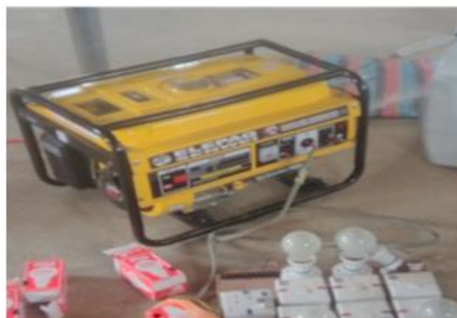
Fig 1:- Test engine and load bank
