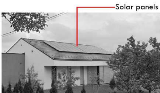
Figure 9.7 Solar panels over the roof tiles
