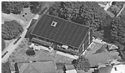
Figure 8.6 Solar panels over the roof tiles
