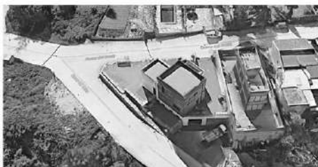
Figure 13.6 Picture of the roof
