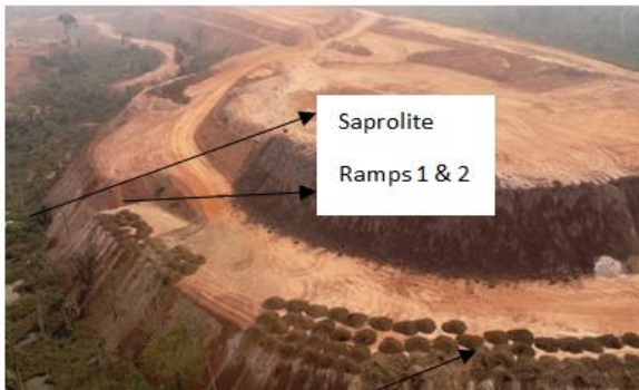
Figure 3: Hill under construction, with sterile saprolite showing the stairway (ramps) layouts.
