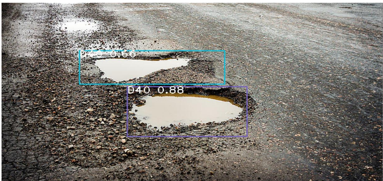
Figure 8: Detected images of Potholes
