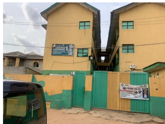
Plate 4: rear view of school. Source: field survey, 2021.
