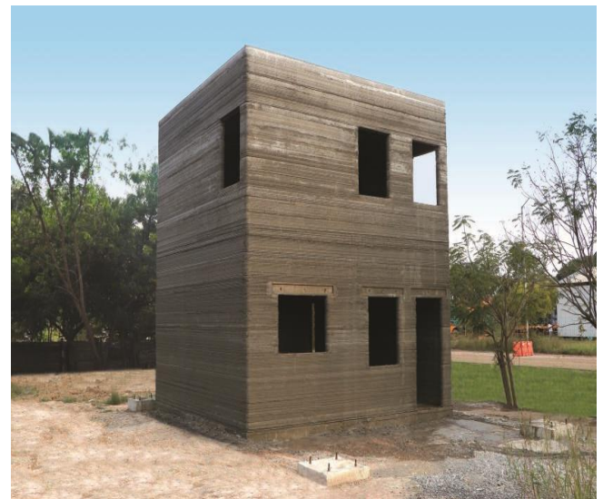
India's first 3D printed two-storey building. Photo via COB
