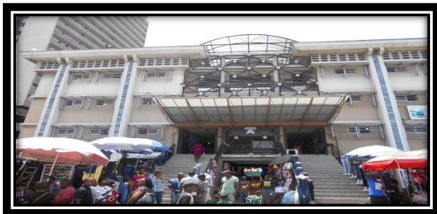
Picture showing external different architectural elements.
