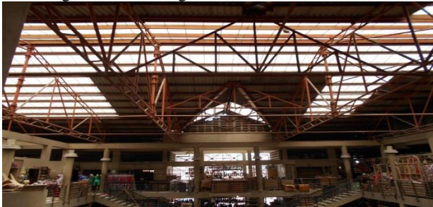
Figure 15 showing the internal roof members.
